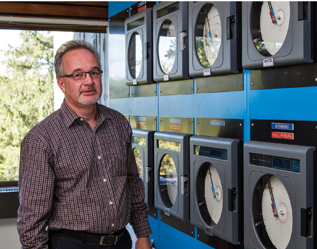
LEFT: Dwight Boyd, the director of engineering with the Grand River Conservation Authority, stands in the control room at the GRCA's main office in Cambridge.
